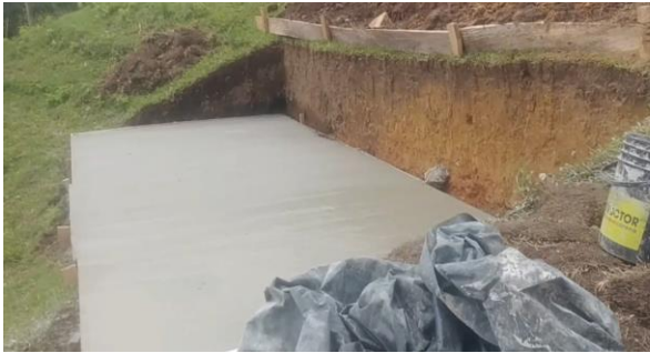
Figure 2: Photograph of water treatment plant construction site.
