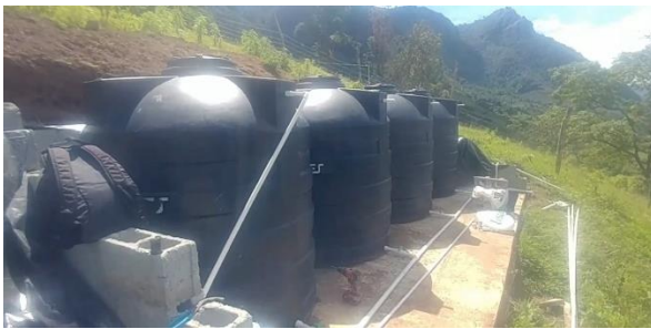
Figure 3: Construction of the water treatment plant.
